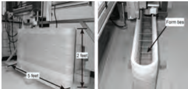
Fig. 2. A concrete wall structure formed by a CC machine, incorporating specially designed reinforcement ties inserted by hand between the layers.
