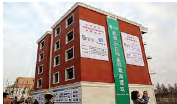
(b) A structure built using 3D printing [5].
