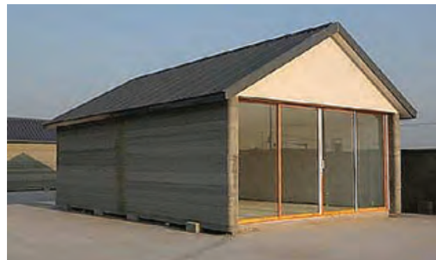
Fig. 1 (a) Win Sun's first 3D-printed home (2014) [5]
